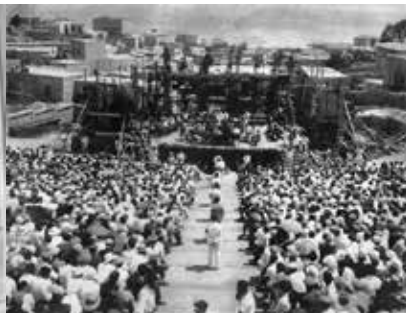
Workers’ House with amphitheatre, which was built by Phillip Böhm, member of Tchelet Lavan in Haifa (source: Historical archive Technion, Haifa)
